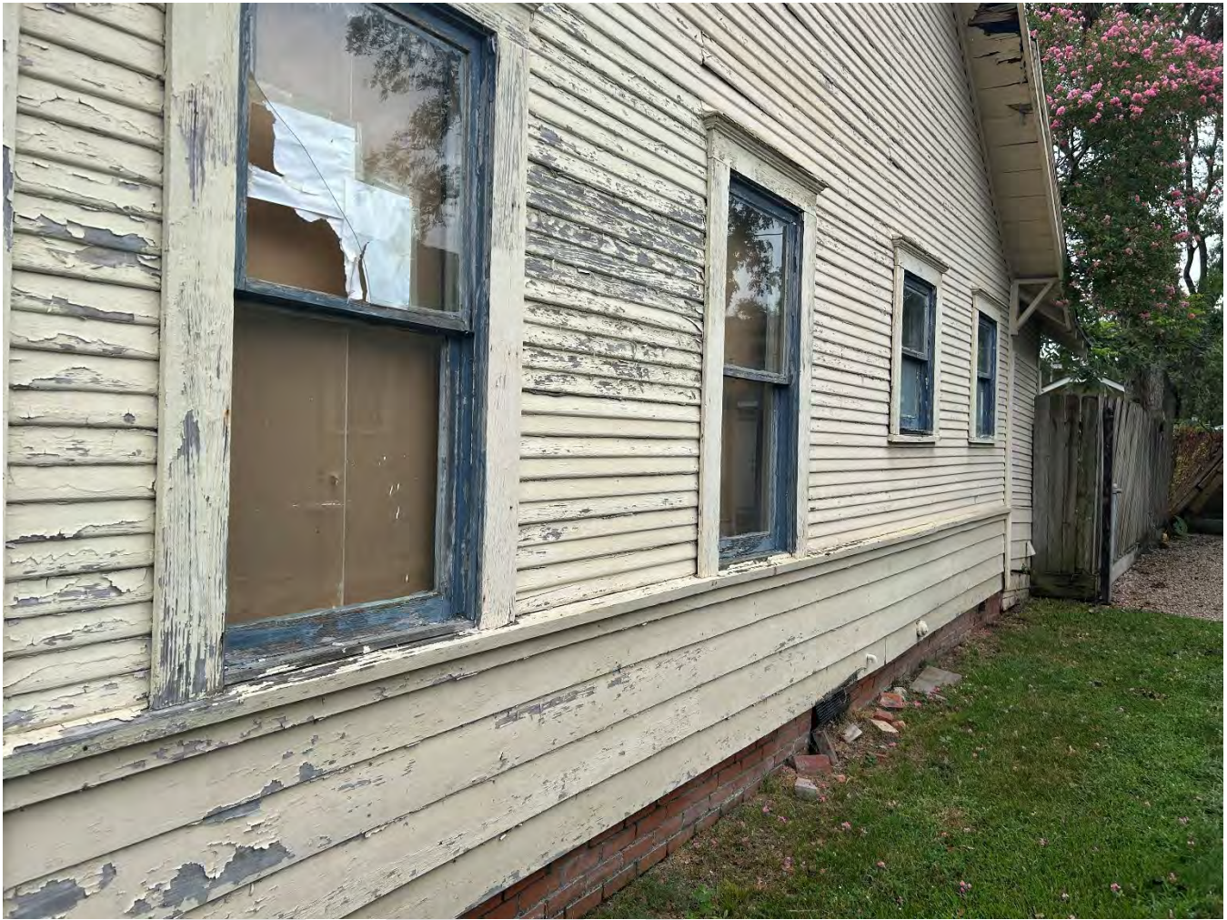
Figure 6 - Staff Photo West Elevation
