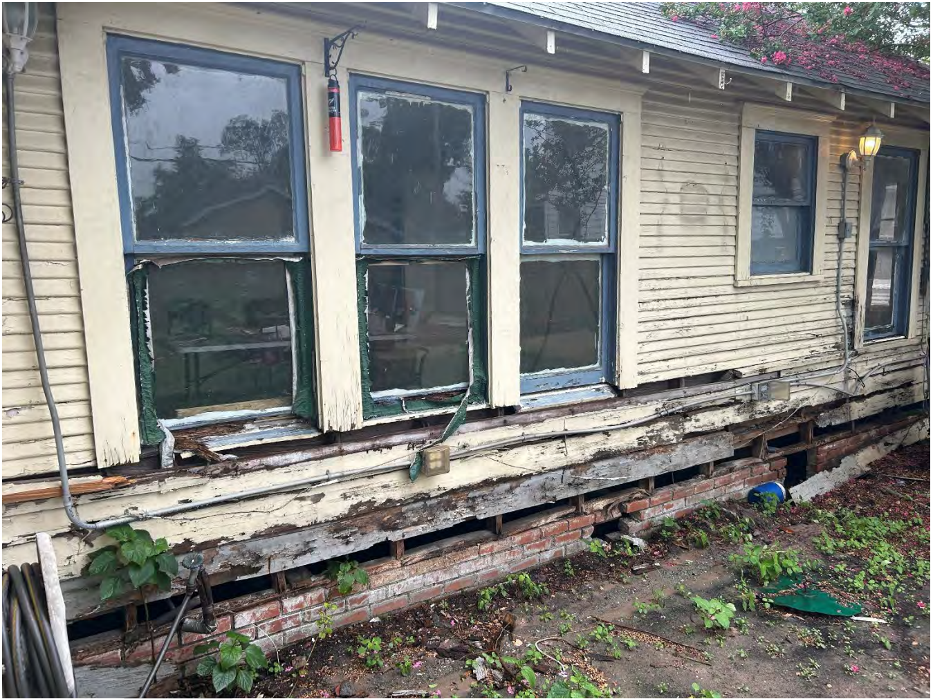
Figure 9 - Staff Photo Rear Elevation Partial
